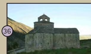
36 Sant Serni de Cabó: A highly modified Romanesque church with an original chancel that was initially trefoil and faced west. The temple was built in the 11th century and reformed in the 17th or 18th century.
